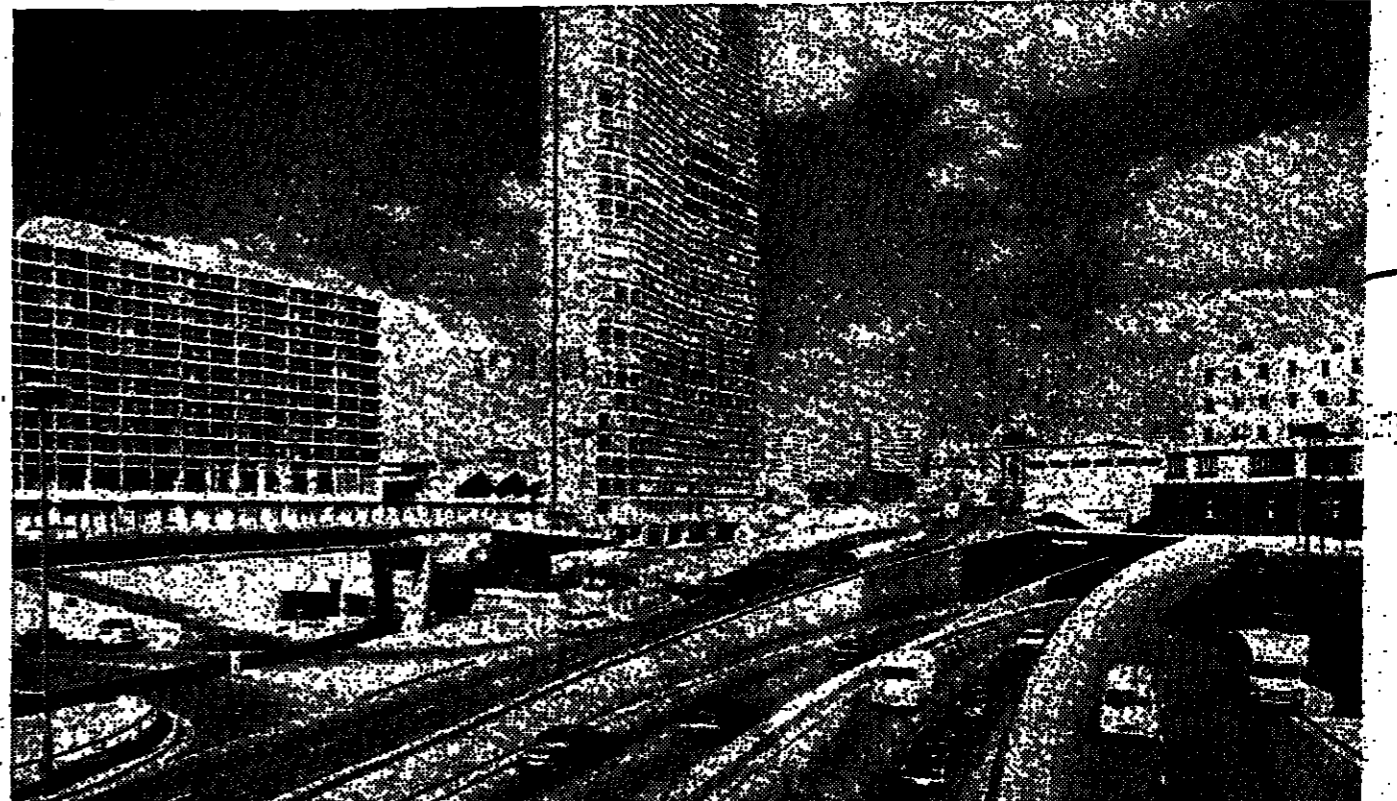
Example of what has been happening on a larger scale around Birmingham. On a main route that takes in the recently built Castle Vale housing scheme, and which has attracted a lot of warehousing and similar projects, as well as a hyper-
